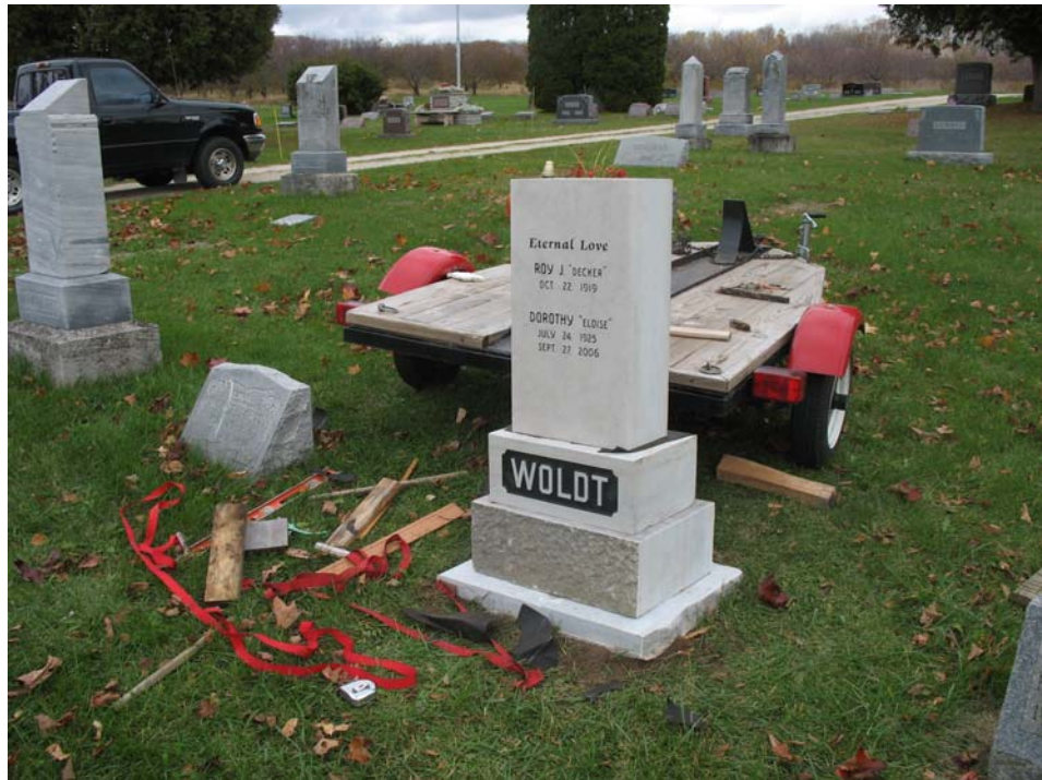
By positioning the trailer on the uphill side, I was able to slide, roll, and tilt stones into place.
